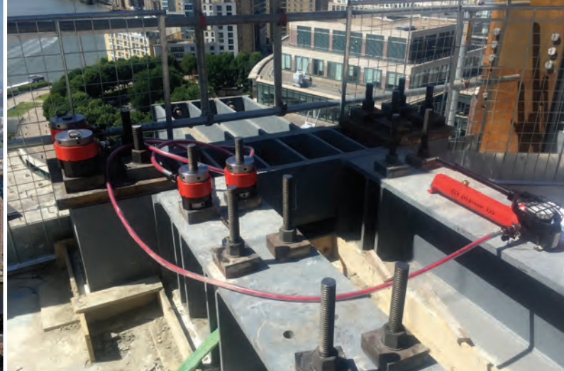
Figure 7: Tensioning of TC tie bracket.
