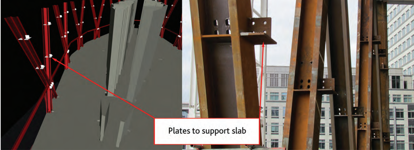
Figure 4: Edge supports for PT slabs.
