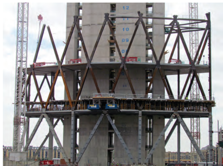
Figure 5: PT slab is installed in between the nodal floors.
