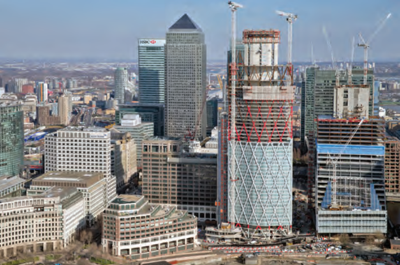
Figure 6: During construction. (Photo: Peter Matthews.)
