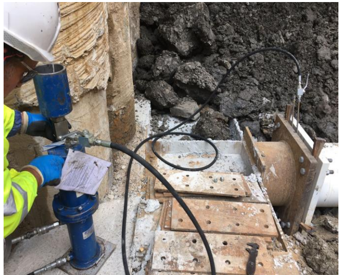
Flat Jacking (pre-loading temporary works)
