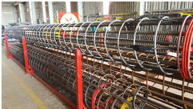
Lifting of Reinforcement Cages
