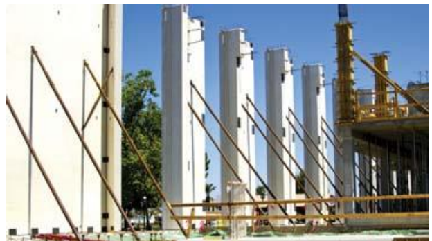
Propping Precast Walls and Columns
